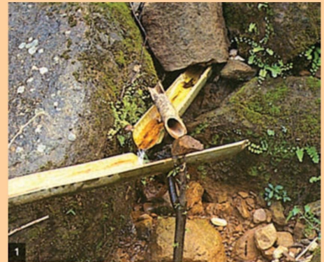
Picture 1: Bamboo pipes are used to divert perennial springs on the hilltops to the lower reaches by gravity.
