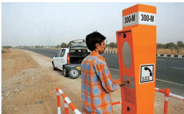
Fig. 7.10 : Emergency call box on NH-48
