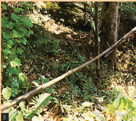
Picture 2 and 3: The channel sections, made of bamboo, divert water to the plant site where it is distributed into branches, again made and laid out with different forms of bamboo pipes. The flow of water into the pipes is controlled by manipulating the pipe positions.
